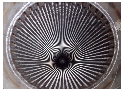
24 in. screen installed
